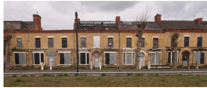
Figure 18.1 : Exterior perspective of initial site conditions prior to construction
