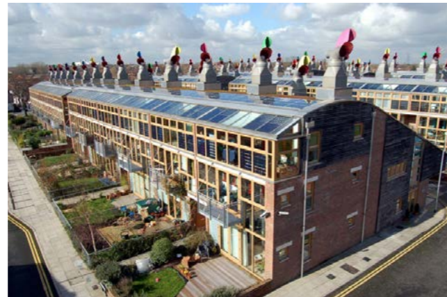
Figure 16.1 : Exterior perspective of BedZed Eco Village development
